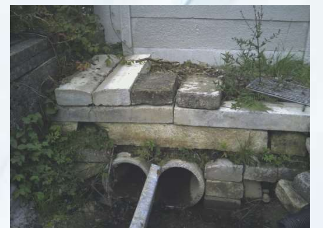
View of inlet structure to be replaced
